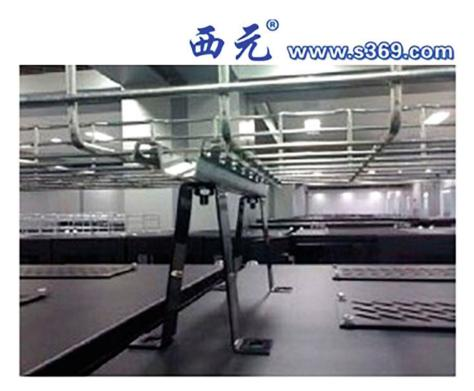
Fig. 2.64 Installation of supporting bridge for rack
