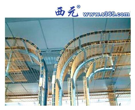
Fig. 2.63 Layered installation of bridges
