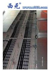
Fig. 2.66 Cabling channels under the raised floor
