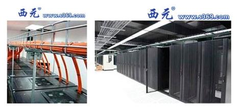
Fig. 2.67 Ceiling-mounted cabling channels
